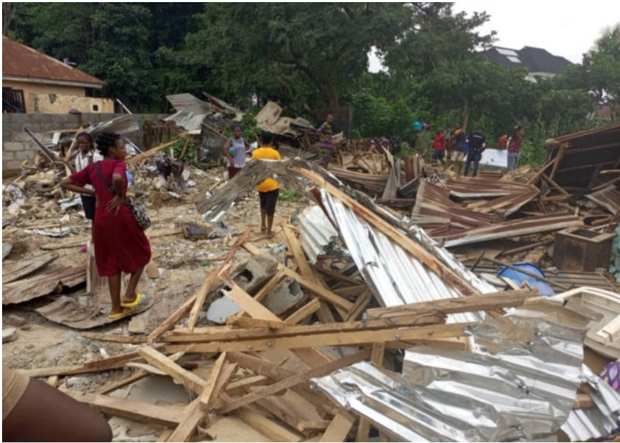
Demolition at Durumi 3, an indigenous community in the FCT, on August 17, 2022
