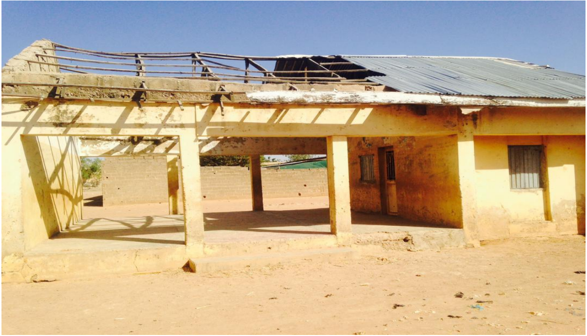
Pic. 5: Zara PHC Building, Kumbotso LGA, Kano
