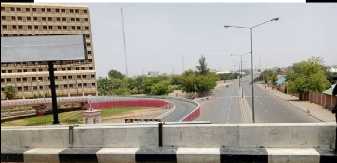
The ever-busy Kofar Nassarawa Flyover overlooking the equally busy Ibrahim Taiwo Road, looking deserted while Kano was under the lockdown Photo: TheCable
